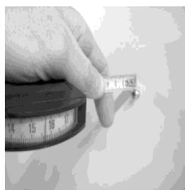
3. LA VIS DOIT DEPASSER DU MUR DE 8 MM MAXIMUM
