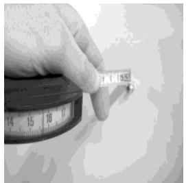
3. LA VIS DOIT DEPASSER DU MUR DE 8 MM MAXIMUM
